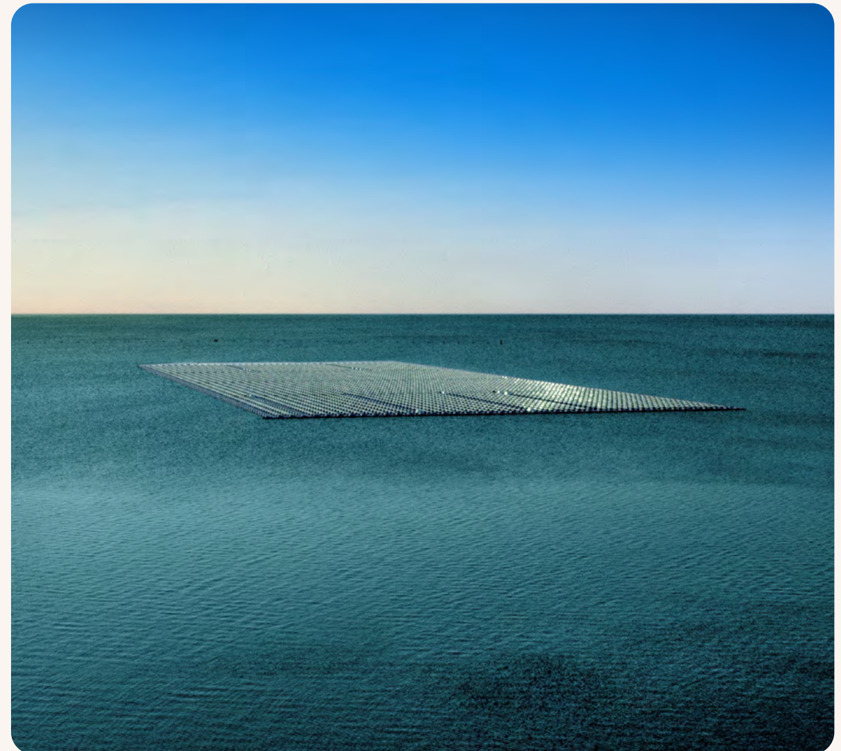
Floating Photovoltaic Solar Platform in Sobradinho – Zeca Teixeira
