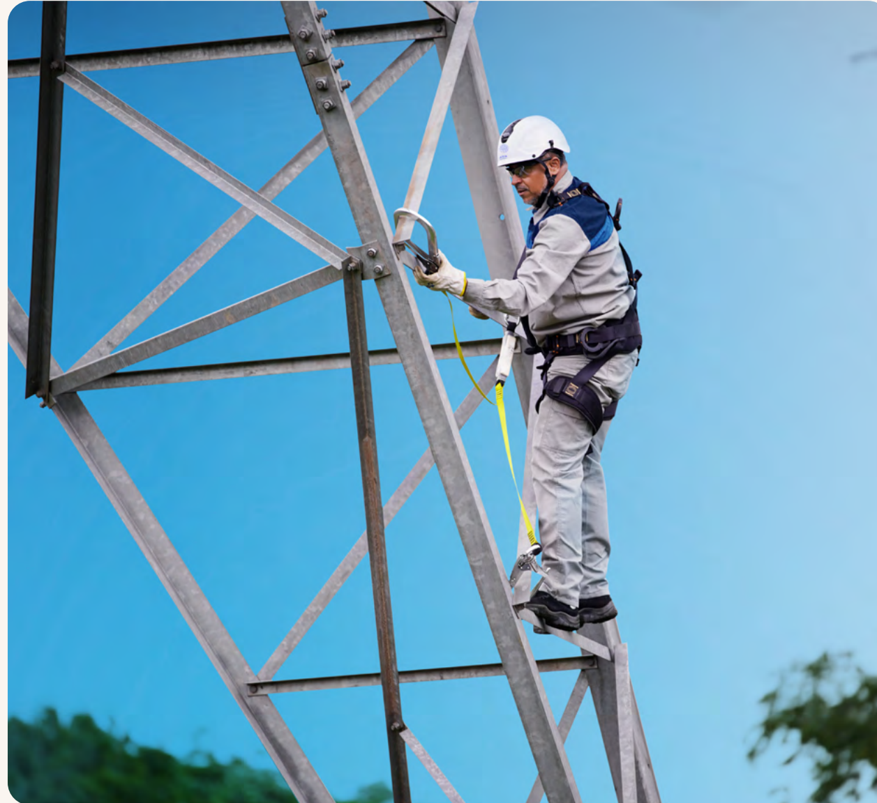
Transmission line maintenance - AXIA Collection
