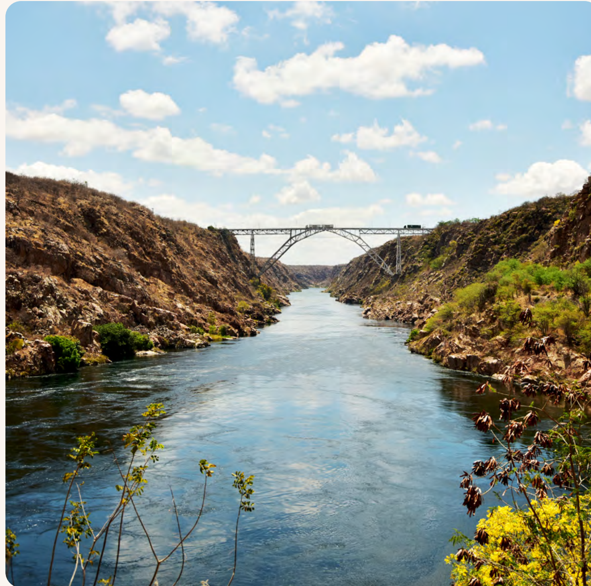
Dom Pedro II Metal Bridge crossing the São Francisco River, located in the Paulo Afonso region, Bahia - AXIA Collection
