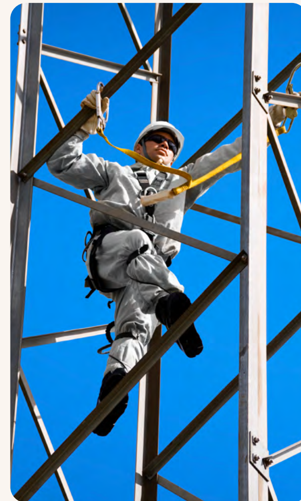
Substation Foz do Iguaçu - AXIA Collection
